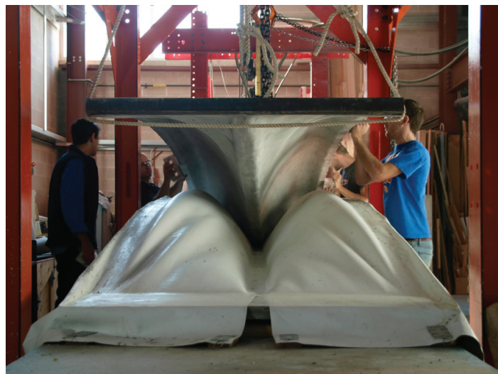
Figure 3. Concrete cast of a vault being lifted made from an inverted fabric formed concrete mould (and modeled in plaster from during the initial study in (Figure 21).
