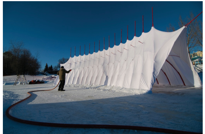
Figure 5. Coar spraying river water onto the fabric skin of the fiberglass framed structure (from Figure 1). The structure acted as a skating tunnel for the Warming Huts Competition in Winnipeg, Manitoba in 2011.
